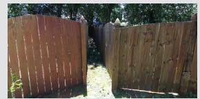
Back-to-back fences can trap debris between them, creating a susceptible fuel bed for embers to ignite both fences. The two fences together provide greater fuel for a more intense fire.
